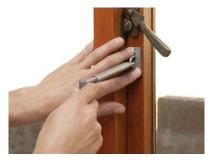
3. Check that the window or door opens and closes and adjust if required
