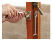
8. Insert the four one-way screws
